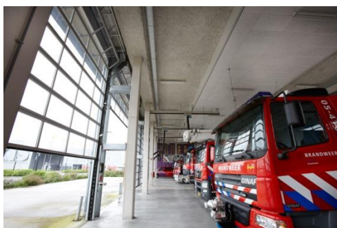
Fire station Enschede - Netherlands
